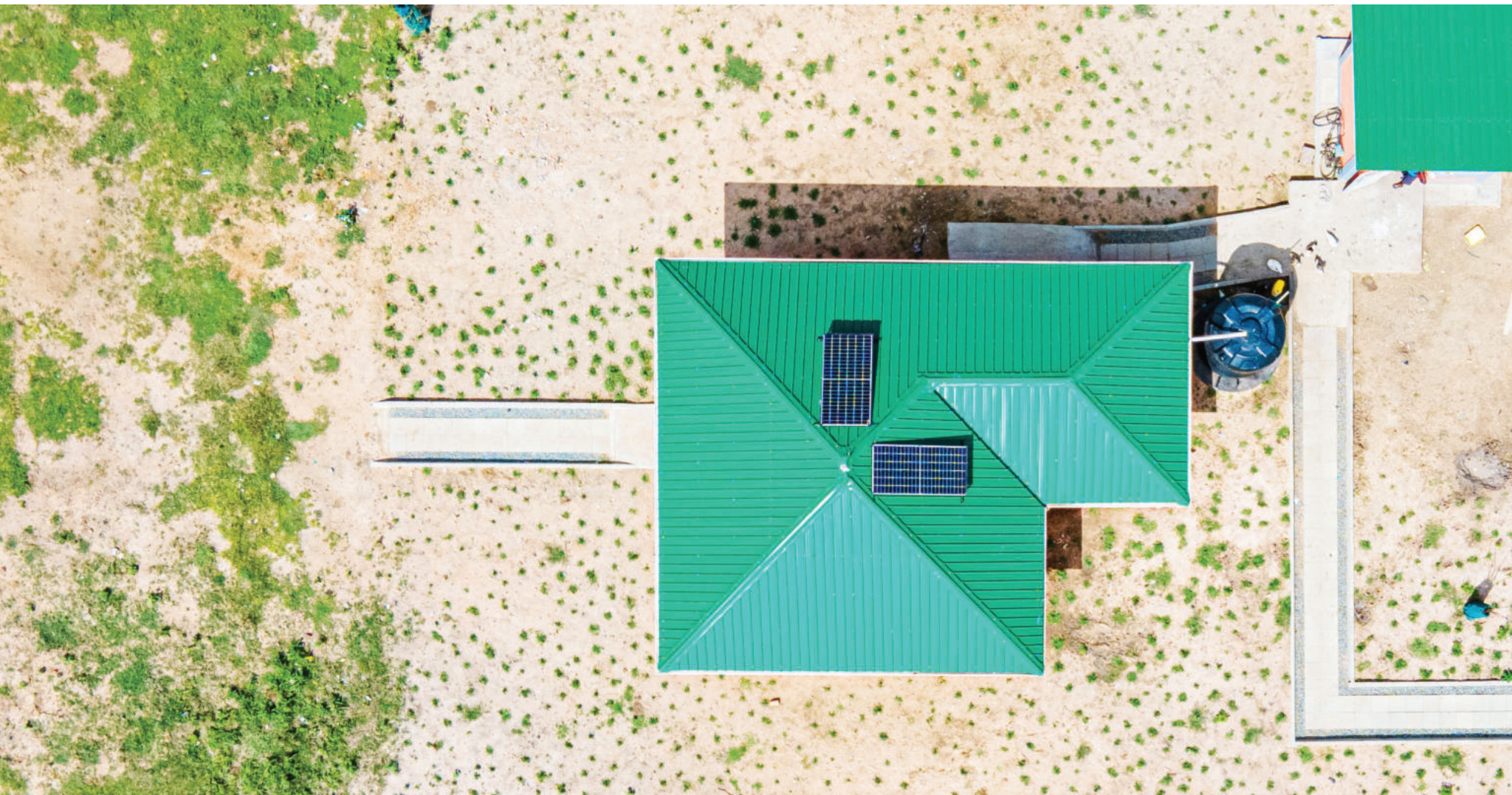
▶ Resettlement houses for project affected persons whose primary residence was affected by the Tilenga project land take
