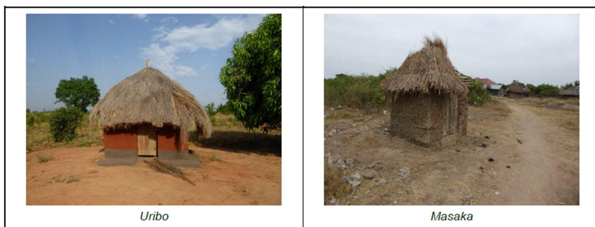
Figure 16-24: Covered Pit Latrines
