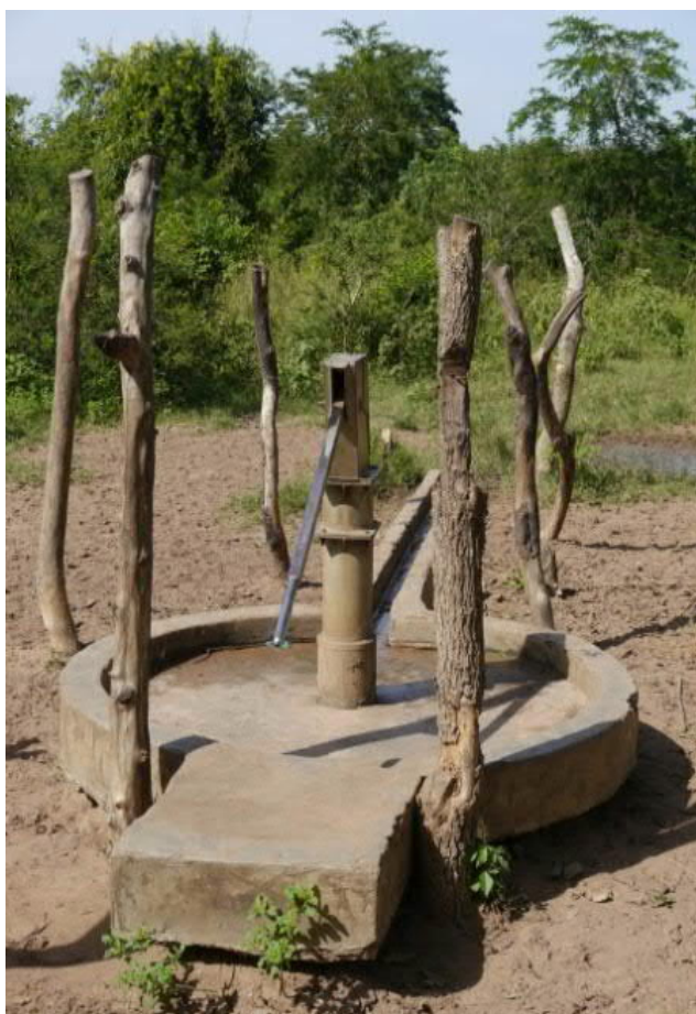
Figure 19-15: A hand pump near Well pad NGR-01
